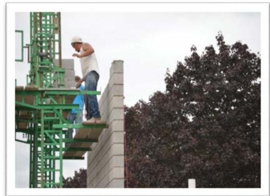
Pump jacks consist of a platform supported by moveable brackets on vertical poles.
