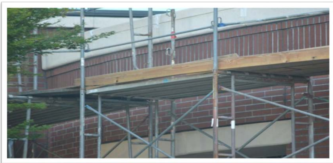
Frame scaffolds are the most common type of scaffold because they are easy to use.
