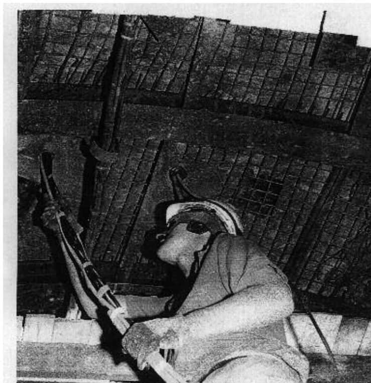
Installing a cablebolt in an arched roadway (photograph courtesy of Pozament Ltd)
