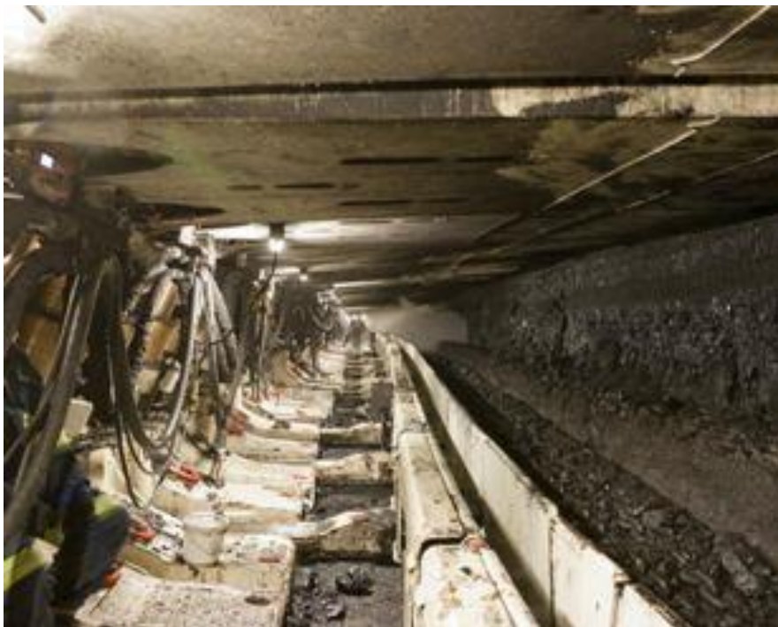
Figure 58. Picture of a completed longwall panel setup (Mining World, 2008).
