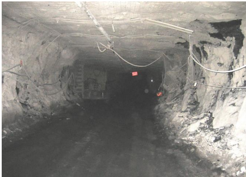
Figure 16. Use of a crib in a crosscut along a haulage way. (Klemetti, 2013)
