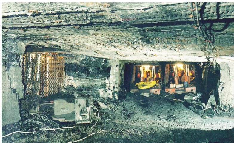
Figure 42. Illustration of mobile roof supports being used for retreat mining.
