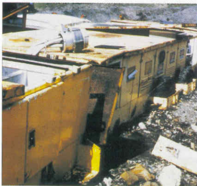
Mine power centers containing PCB capacitors outside an underground Utah coal mine.
