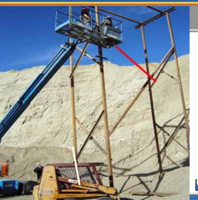
The red line shows the original location of the tubing, the white line shows where it landed, inside the cab.
