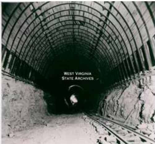
Hawk's Nest Tunnel construction, West Virginia, 1930-1931. Source: West Virginia Photos database.
