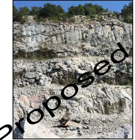
On Soptember 8, 2016, a 58-year old Haul Truck Operator with 23 years of experience was killed at a granite mine. The victim was operating a Caterpillar 773E haul truck and was returning to the pit to be loaded with shot rock. The truck veered from the right side of the haul road to the left and traveled over the berm at the top of the highwall. The truck landed upside down approximately 150 feet below. The victim was found outside the haul truck.
