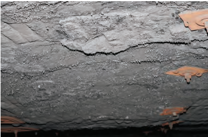
Photo 5. Evidence of coking on mine roof inby the first open crosscut in the #1 Entry. This type of coking is a residue of a coal dust explosion.
