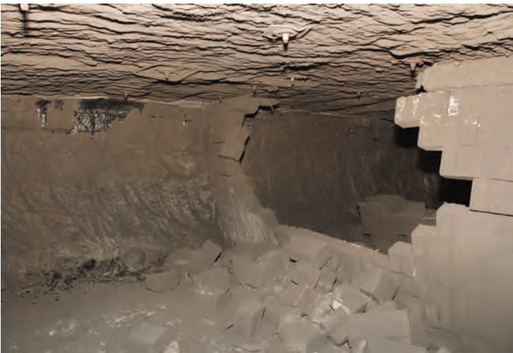
Photo 9. Stopping blown out toward the north as a result of the initial path of forces, at 73 crosscut, northeast of 78 switch.
