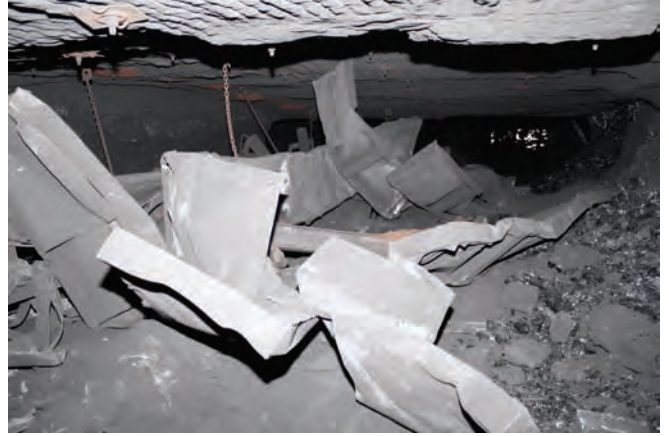
Photo 2. Steel overcast cover panels twisted and crumpled at #1 Crosscut in the Tailgate 22 Section.
