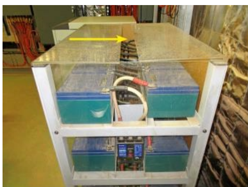
UPS battery cabinets. Left. Potential for inadvertent access as indicated by arrow. Right. Exposed live terminals (arc flash damage indicated by circle).
