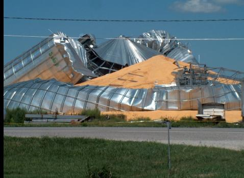
Collapse of a storage bin at East Minot, N.D., Several railroad cars were derailed or buried beneath the grain.
