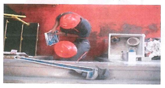
If that tool fell could it strike someone? It probably could. Perform your housekeeping on elevated platforms and scaffold throughout the shift. Don't let scrap material, dust, debris, bolts or tools pile above your toe plate. We can install netting between the toe plate and the top rail to add another level of protection to keep materials from falling to a lower level. Good Housekeeping practices can help us "Stop the Drop".
