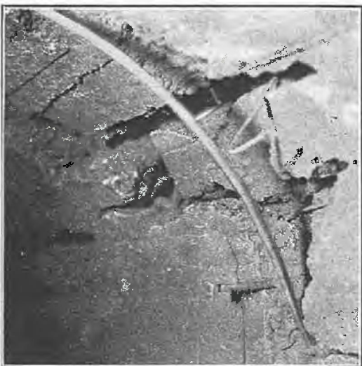
C. REINFORCING ROD PULLED OUT OF CONCRETE IN MAIN GALLERY.
