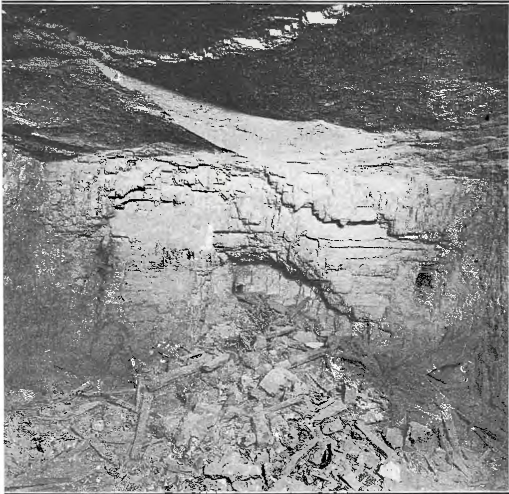
A. SHOT HOLES, AT FACE OF MAIN ENTRY, WHICH CAUSED EXPLOSION; WOOD FRAGMENTS DRAWN INTO CENTRAL CRATER.
