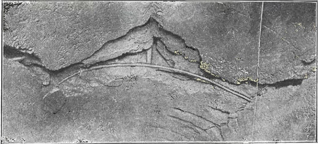
A. RUPTURE IN ROOF OF MAIN GALLERY, EXPERIMENTAL MINE.
