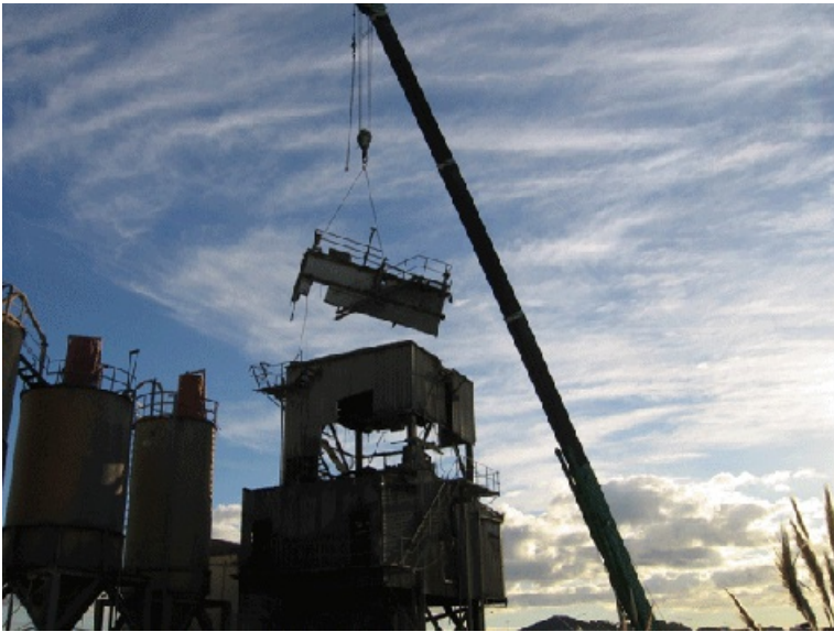
Figure 7: Cut and crane demolition
