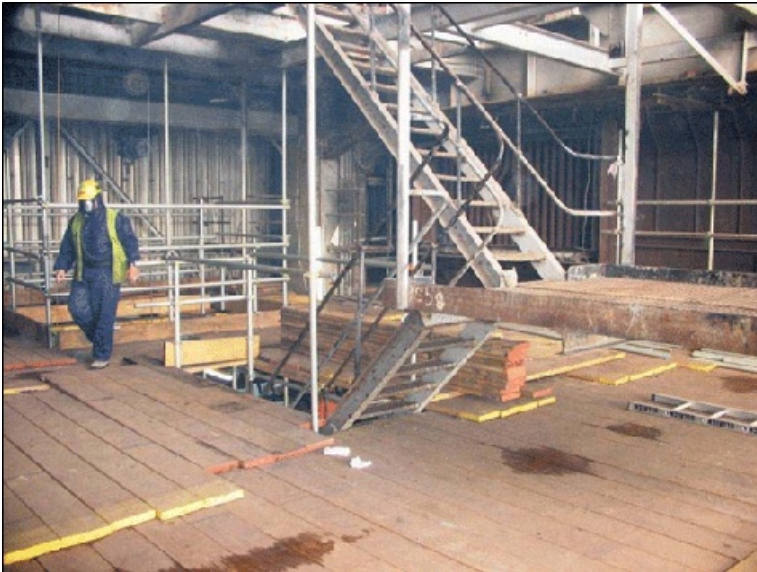
Figure 5: Bird's nest scaffolding used in demolition and asbestos works
