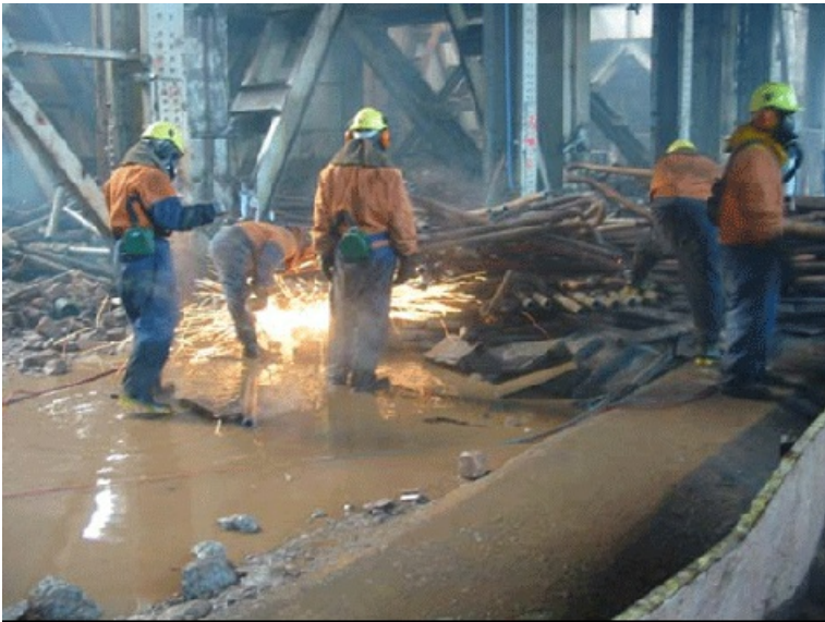
Figure 11: Gas-cutting activity on a demolition site
