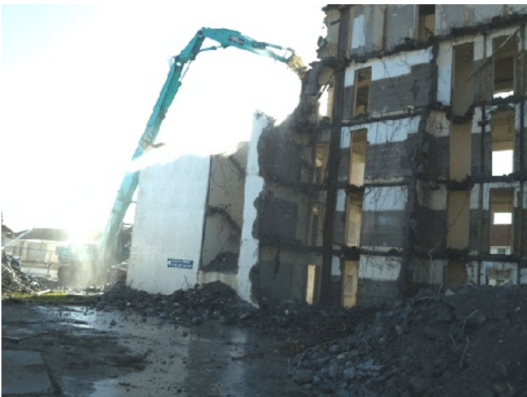
Figure 19: High-reach excavator demolition of multi-storey structure
