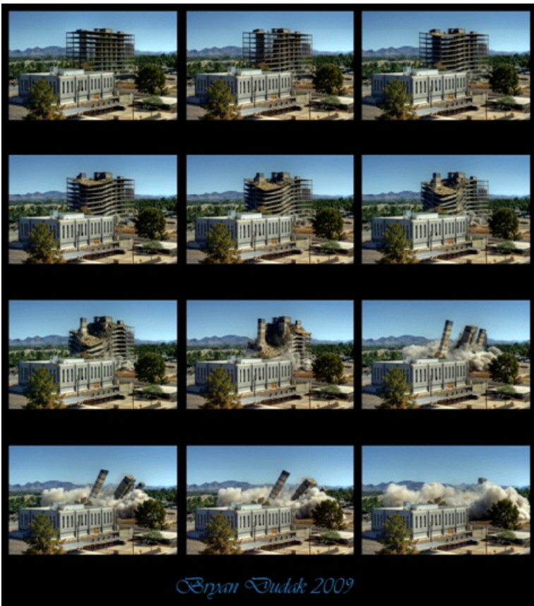
Figure 17: Step-by-step implosion deconstruction (US)
