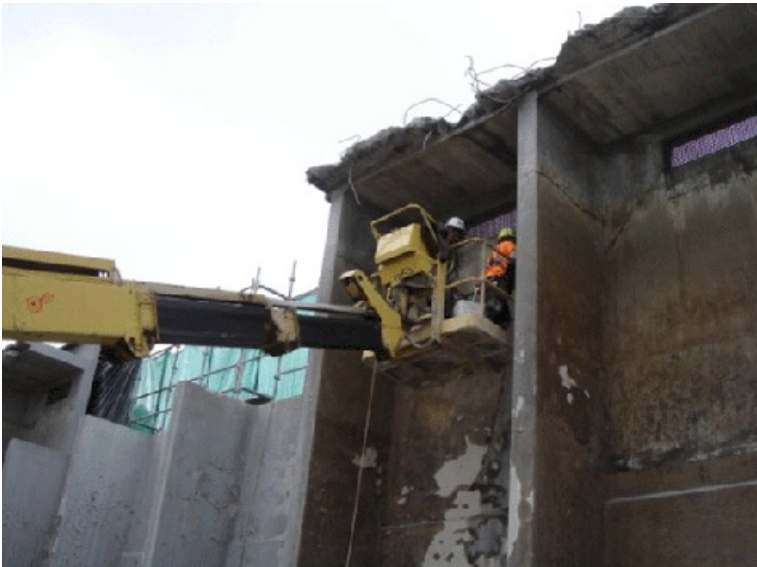
Figure 8: Use of an elevating work platform (EWP) in concrete-cutting demolition
