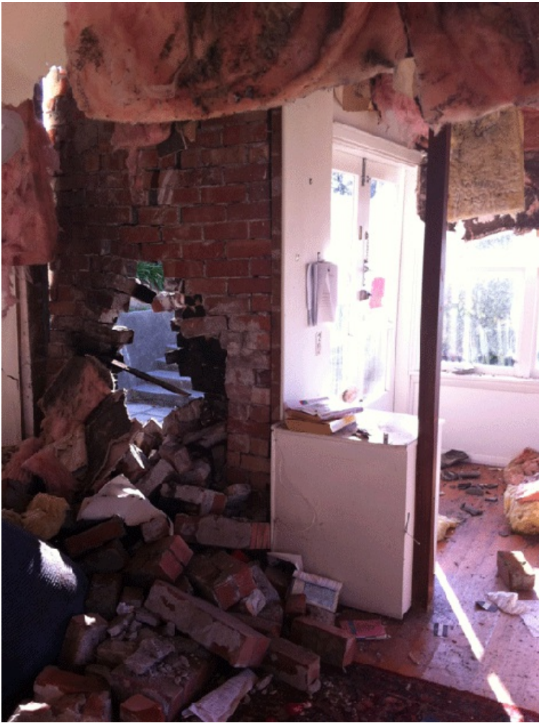
Figure 3: Residential dwelling damaged during the Christchurch earthquake, February 2011
