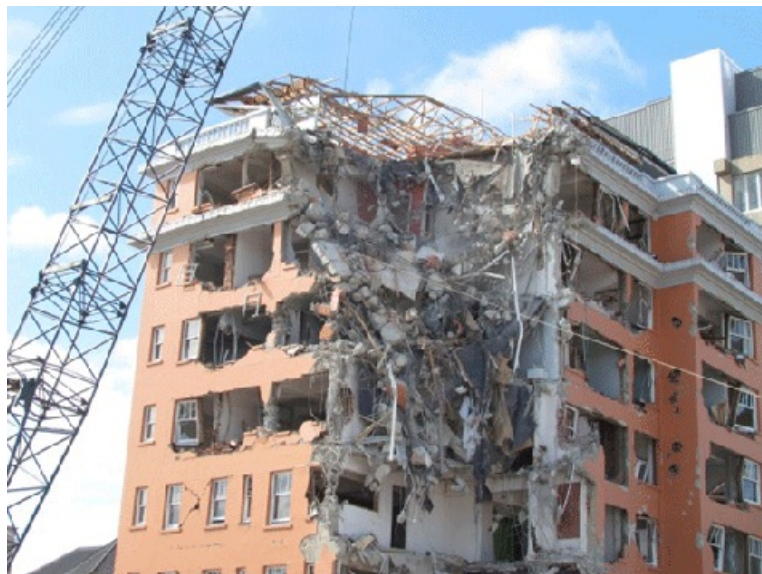
Figure 15: Multi-storey demolition with ball and crane
