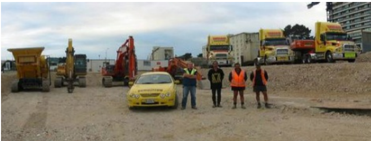
Figure 1: Demolition workers on site in Wellington
