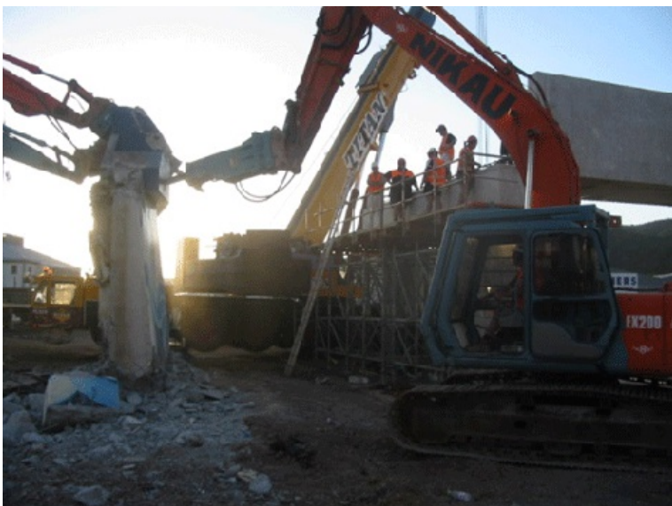
Figure 6: Bridge Pier demolition
