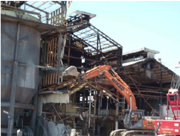
Figure 16: Demolition of silos by pusher arm
