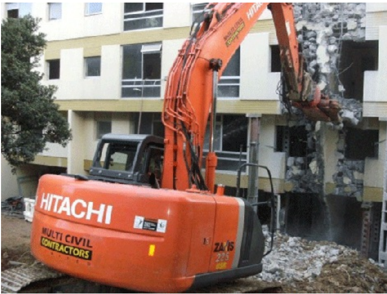
Figure 18: Demolition of reinforced block building by shears
