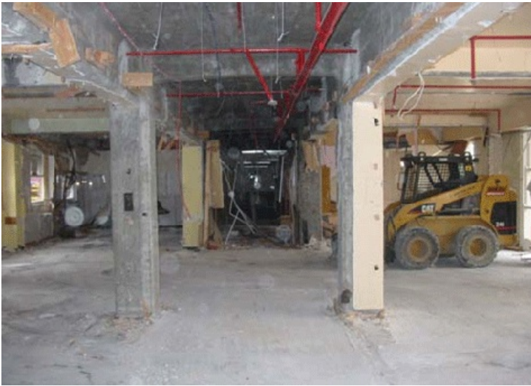
Figure 10: Use of skid steer loaders inside structures
