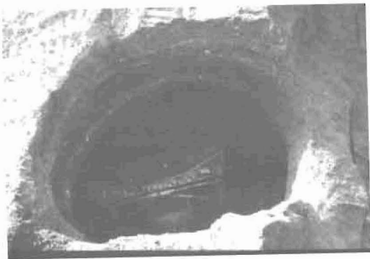
Use extreme caution on surge piles located over draw points.
