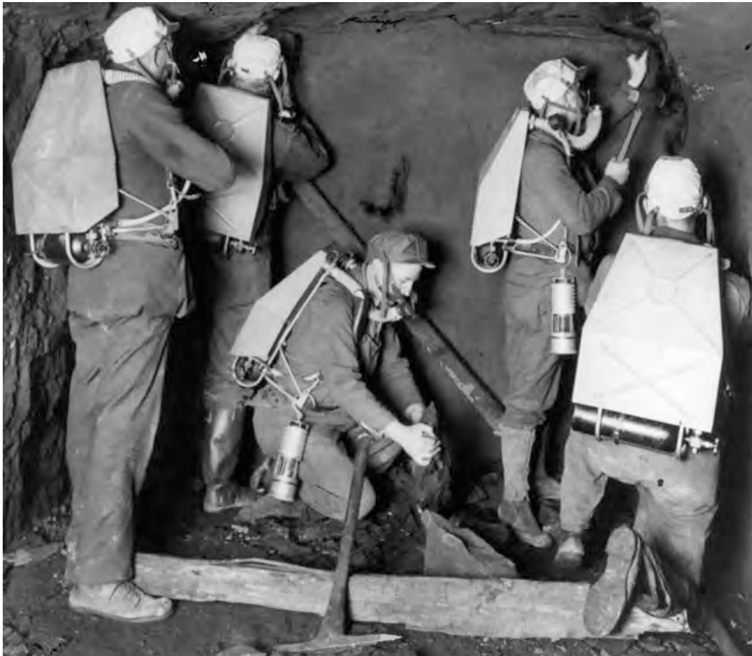
Figure 22. Miners wearing the Gibbs mine rescue breathing apparatus, 1918.
