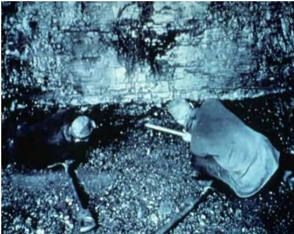
Figure 25. Undercutting coal with a hand pick in the early 20 th century.
