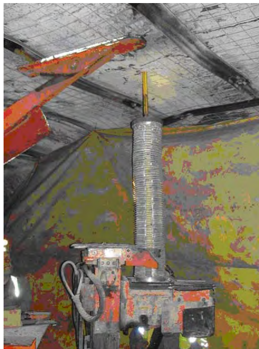
Figure 40. Collapsible Drill Steel Enclosure at start of drilling.
