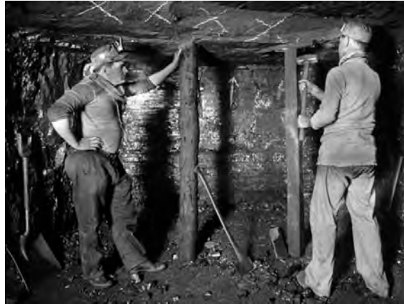
Figure 28. Setting timber posts in a coal mine for roof control.
