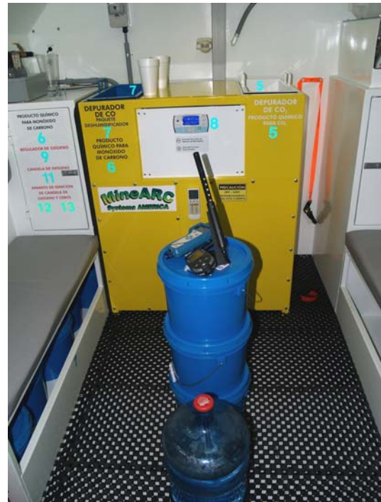
Monitoring equipment placement within refuge chamber
