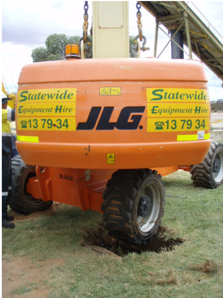
Figure 8 View of crane taking weight and removing boomlift from soak well.
