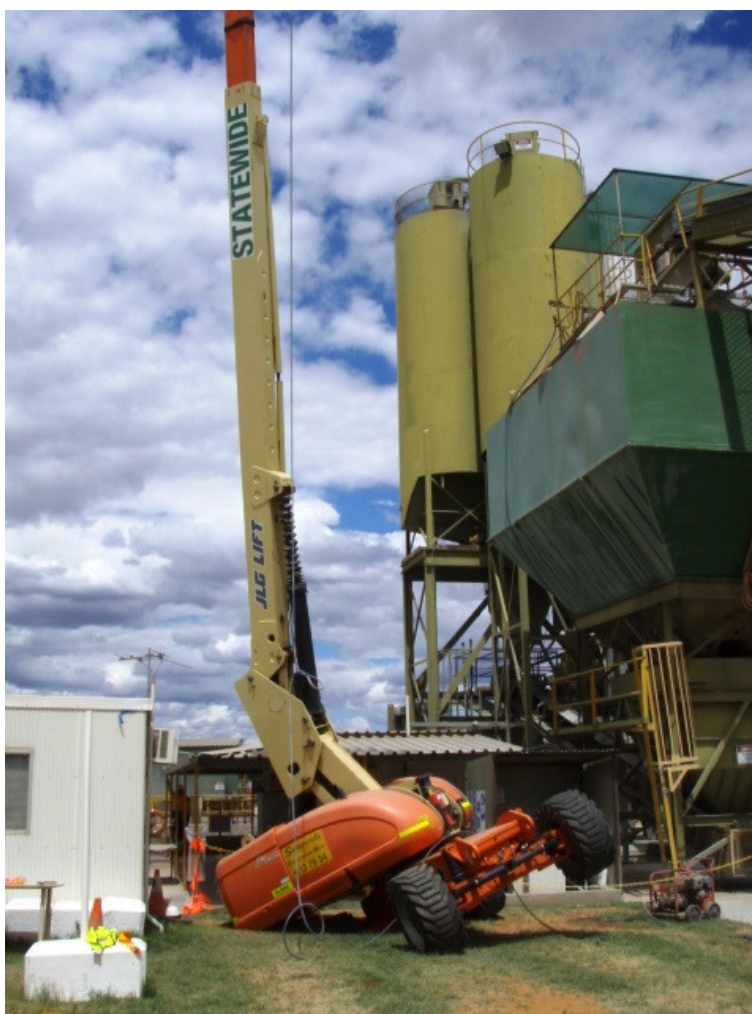
Figure 1 view of work area, workers had completed water blasting conveyer and where moving to silos
