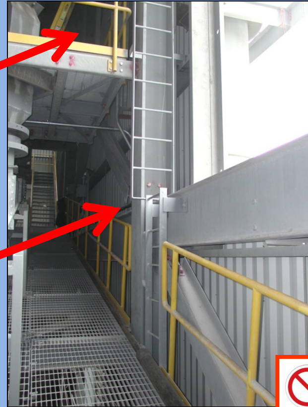
Ladder access and divided ladder sections
