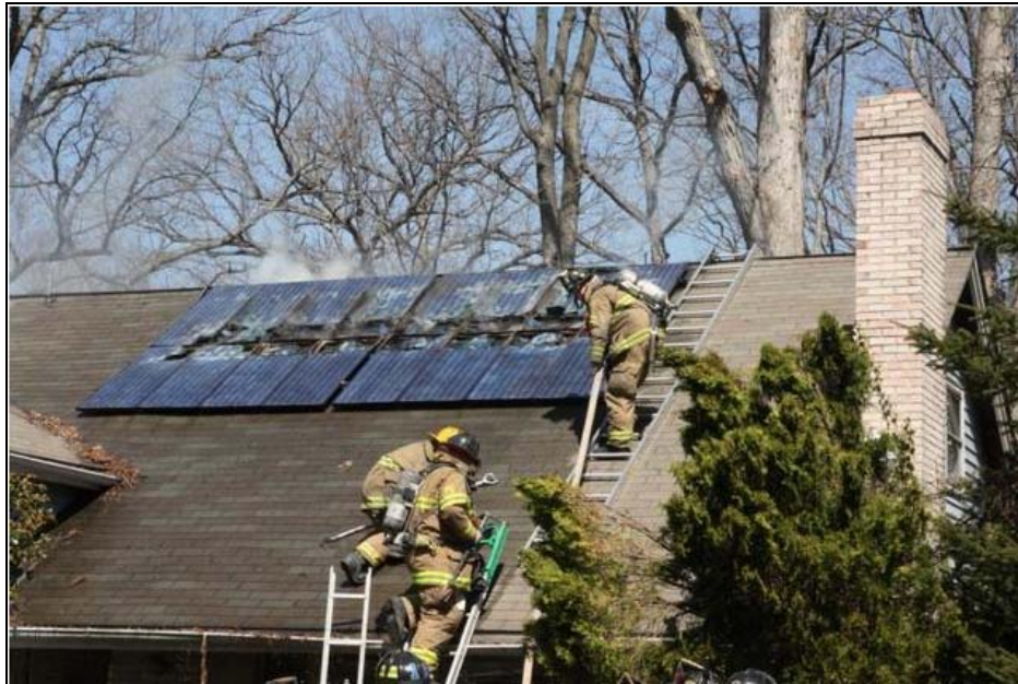
Figure 2-13: Residential PV Fire in March 2010 MD Incident 48
