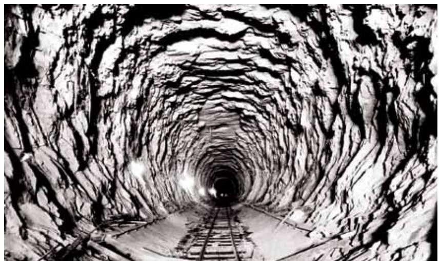
Below: Historical photo of the excavated tunnel
