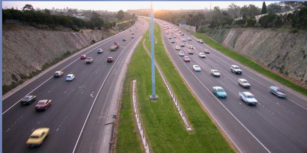
Eastern Freeway, Kew, Melbourne Australia
