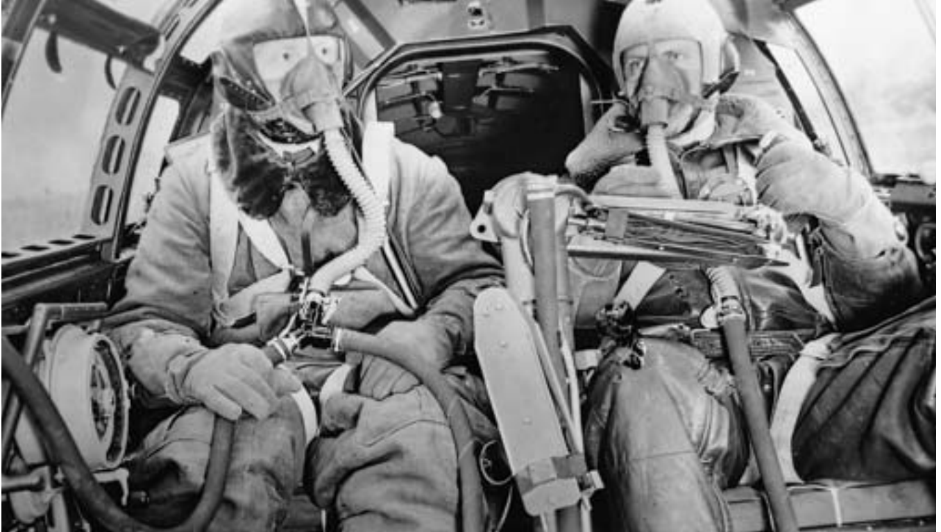
1943 High altitude breathing apparatus for military aircraft. ▲
