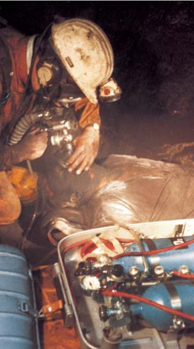
1963 A miner on a rescue mission ▲ with the BG 174 breathing apparatus.
