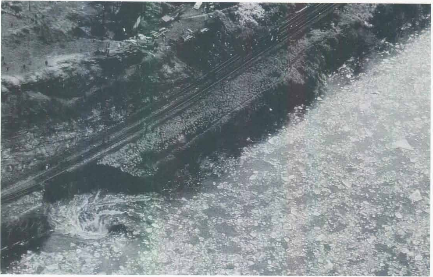
A massive funnel of river water rushes through the collapsed mine tunnel roof. "Water poured down like Niagara Falls," assistant foreman John Williams later testified. Some did not escape the torrent. Twelve trapped men died in the disaster caused by unsafe mining practices.
