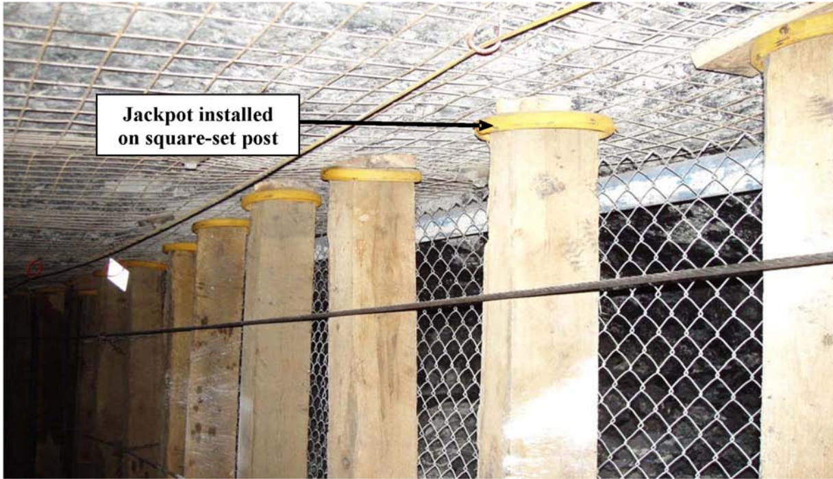
Figure 5 - Hardwood Posts Installed with Jackpots in No. 1 Entry
