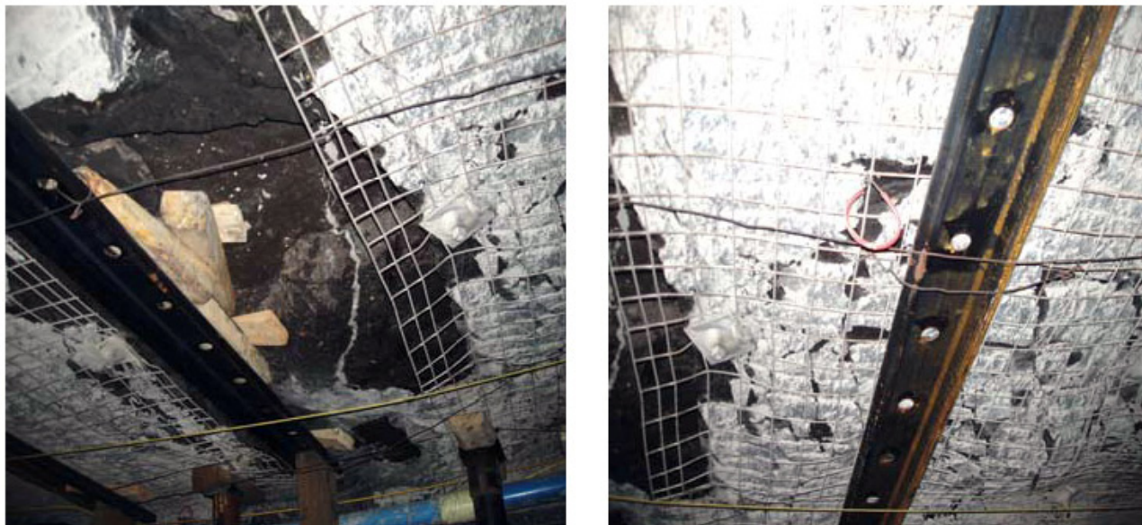
Figure 9 - Steel Channels Installed in No. 1 Entry to Support Deteriorated Roof
