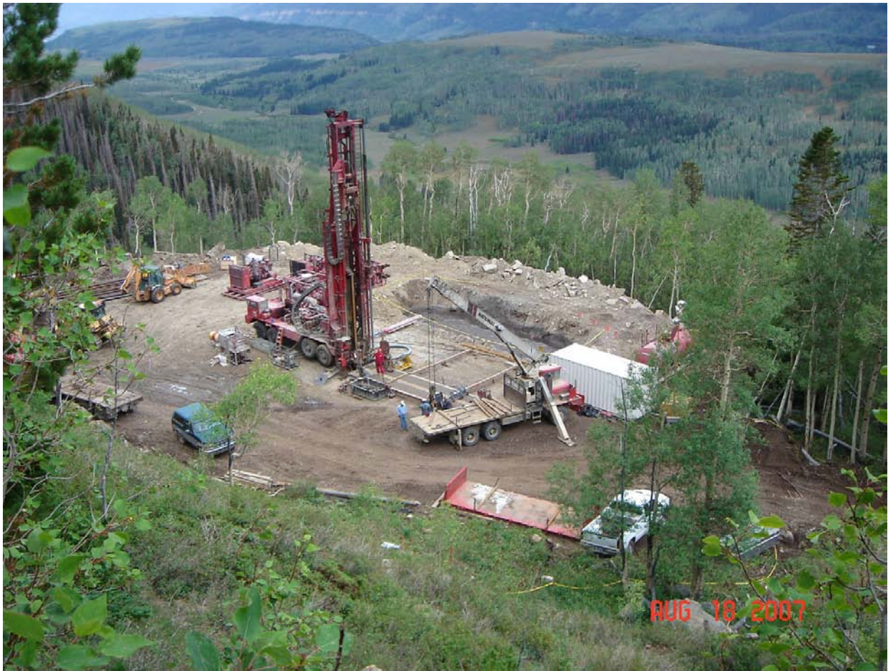
Figure 18 - Drill Rig at Borehole No. 4
