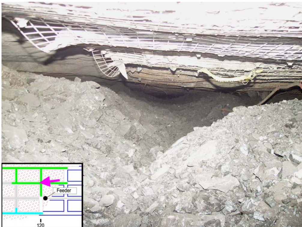
Figure 4 - View of No. 3 Entry after August 7 Burst Entry cleaned by diesel loaders refilled with rubble (view indicated by arrow in index map insert).
