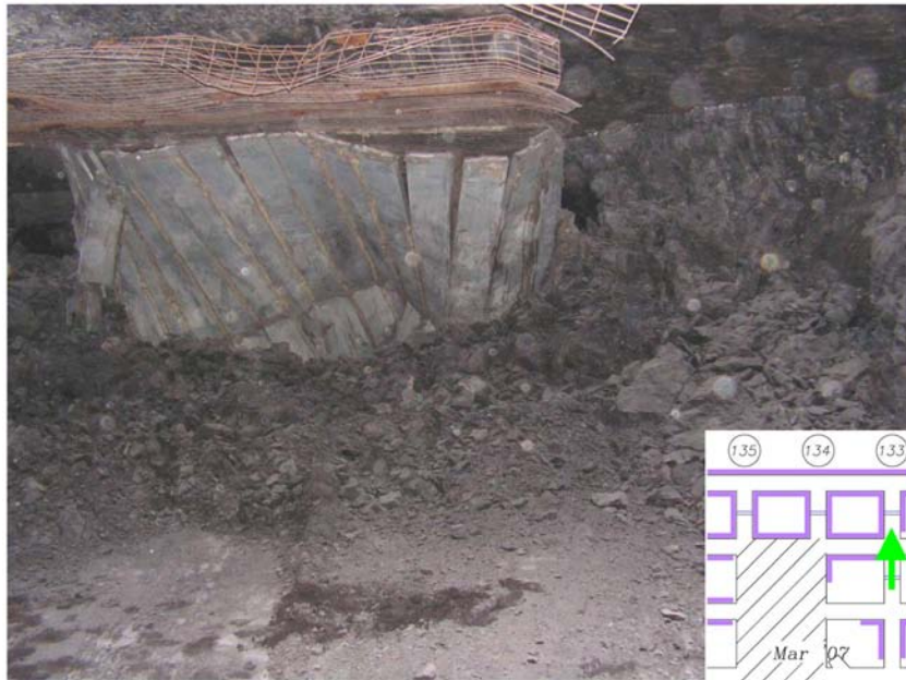
Figure 38 – Stopping Damaged during March 2007 Coal Outburst Accident on North Barrier Section
