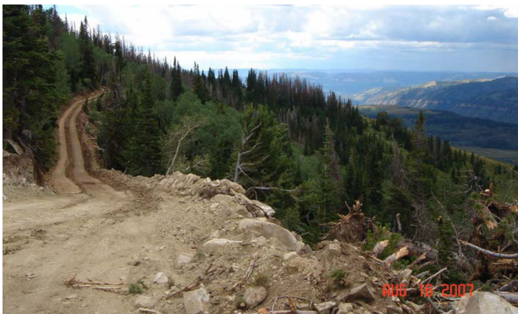
Figure 16 - Mountainous Terrain where Roads and Drill Pads were Constructed
