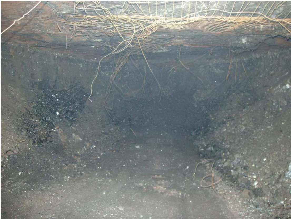
Figure 10 - No. 1 Entry Packed with Coal Rubble Inby Crosscut 124
