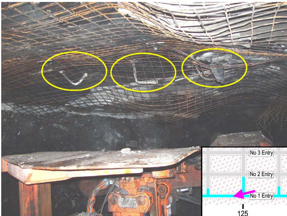
Figure 8 - Damaged Roof Bolts in No. 1 Entry after August 6 Accident Resulting from Northward Movement of Southern Barrier. Mesh shown was installed during rescue operations, over damaged original roof bolts. Camera view is indicated by arrow in index map insert.
