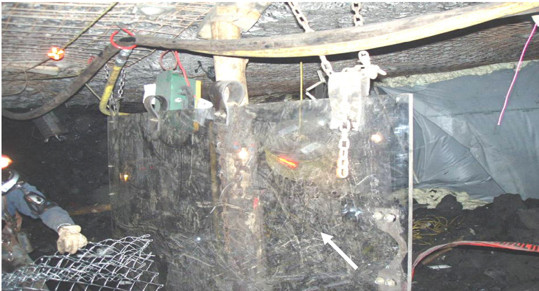
Figure 90 - Sheet of Lexan Suspended from Mine Roof
