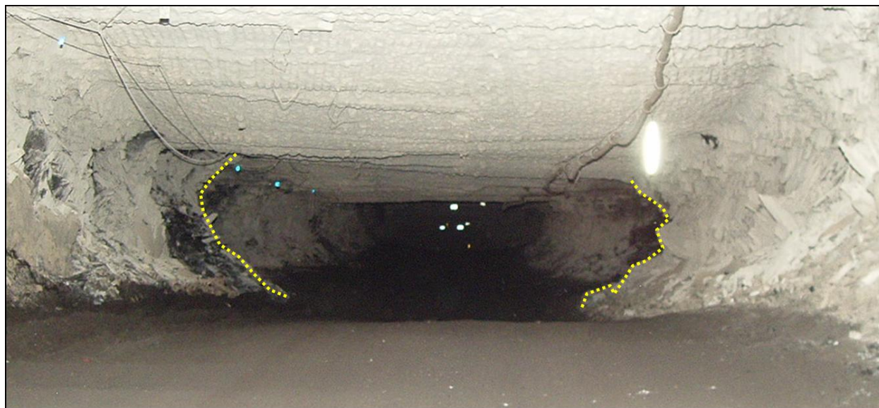
Figure 24 - Hour Glass Shape of Stressed Pillars
