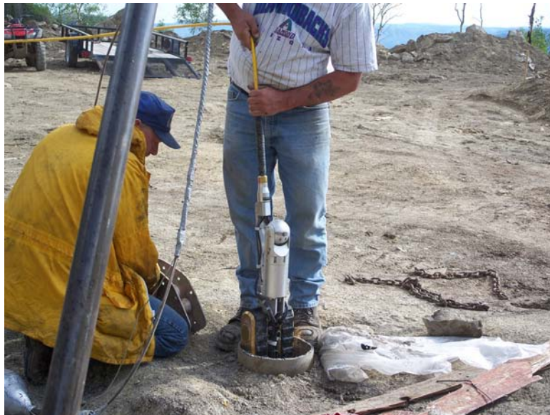
Figure 22 - Robot Being Lowered Into Borehole
