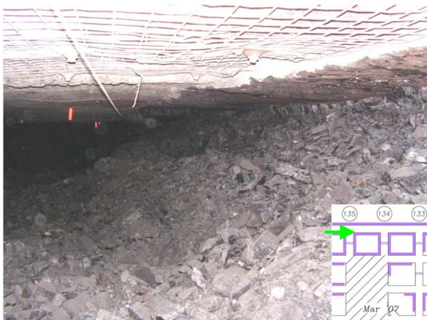
Figure 39 –Damage in No. 4 Entry after the March 2007 Coal Outburst Accident on North Barrier Section
