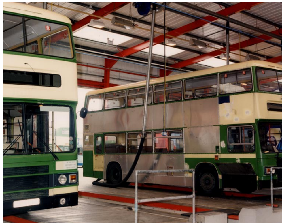
Figure 2 Bus using a tailpipe exhaust extraction system to control emissions
