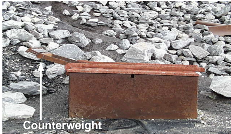
Figure 26.—Counterweight installed to facilitate opening of vault.
