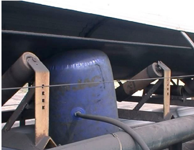
Figure 22.—Using an air bag to lift a conveyor belt.
