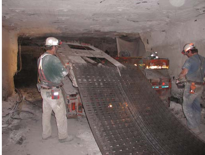
Figure 32.—Use of a winch to facilitate loading roof screen.
