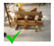
Pipe spool supported by wood must be properly arranged in "square type" manner to have stability and load is distributed
